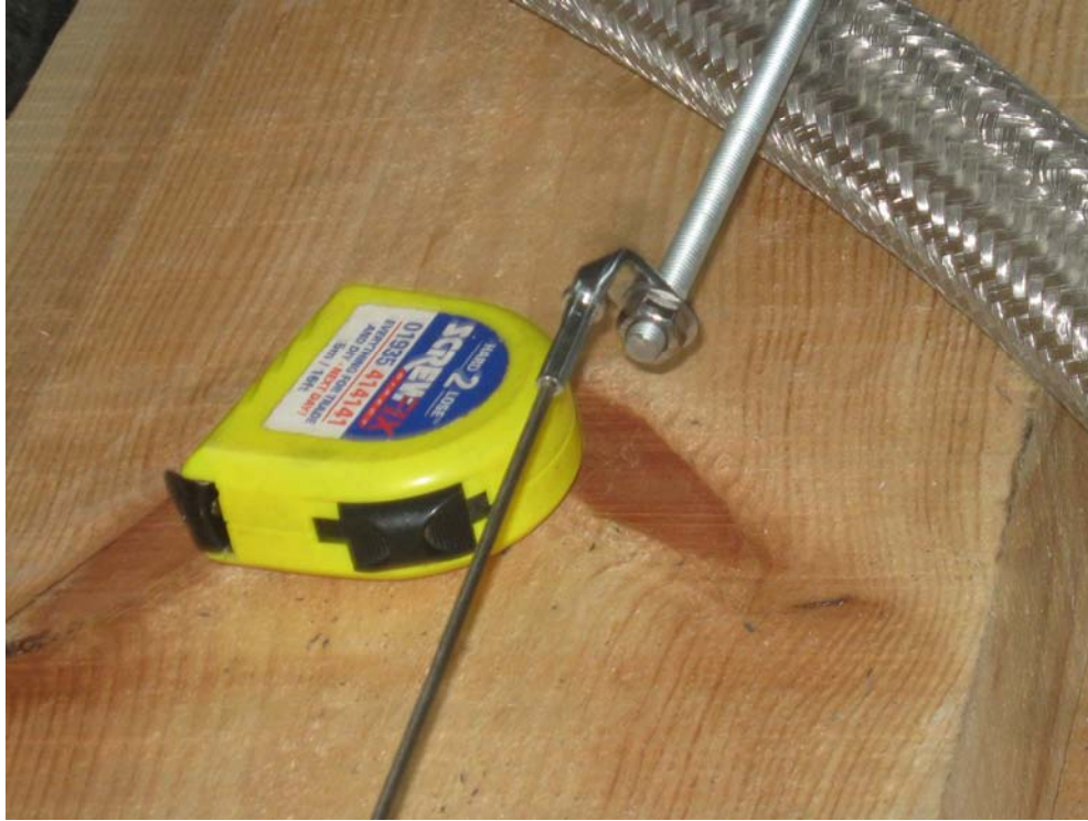
Figure 3 90° eyelet end fixing connected to M8 stud
