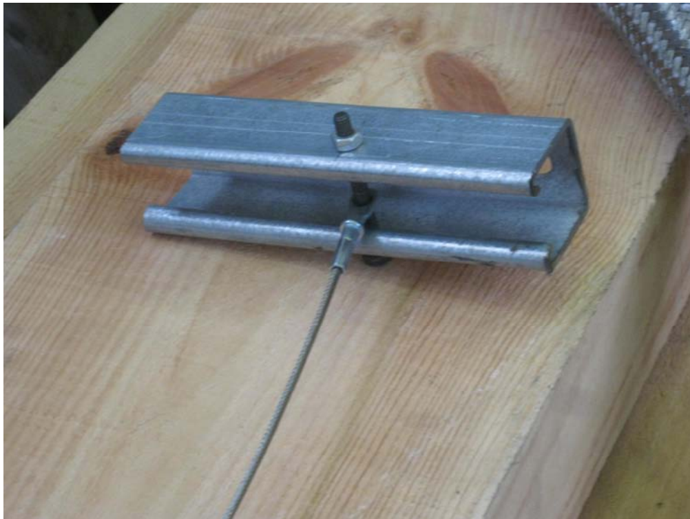
Figure 4 Straight eyelet end fixing connected to channel
